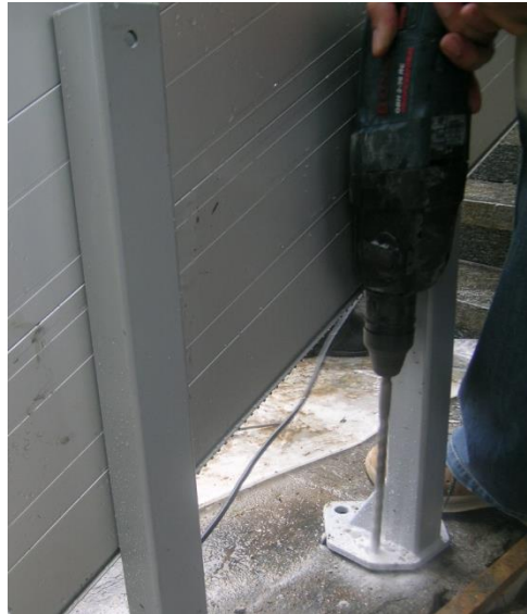
Fig. 9 – Securing the feet to the floor
