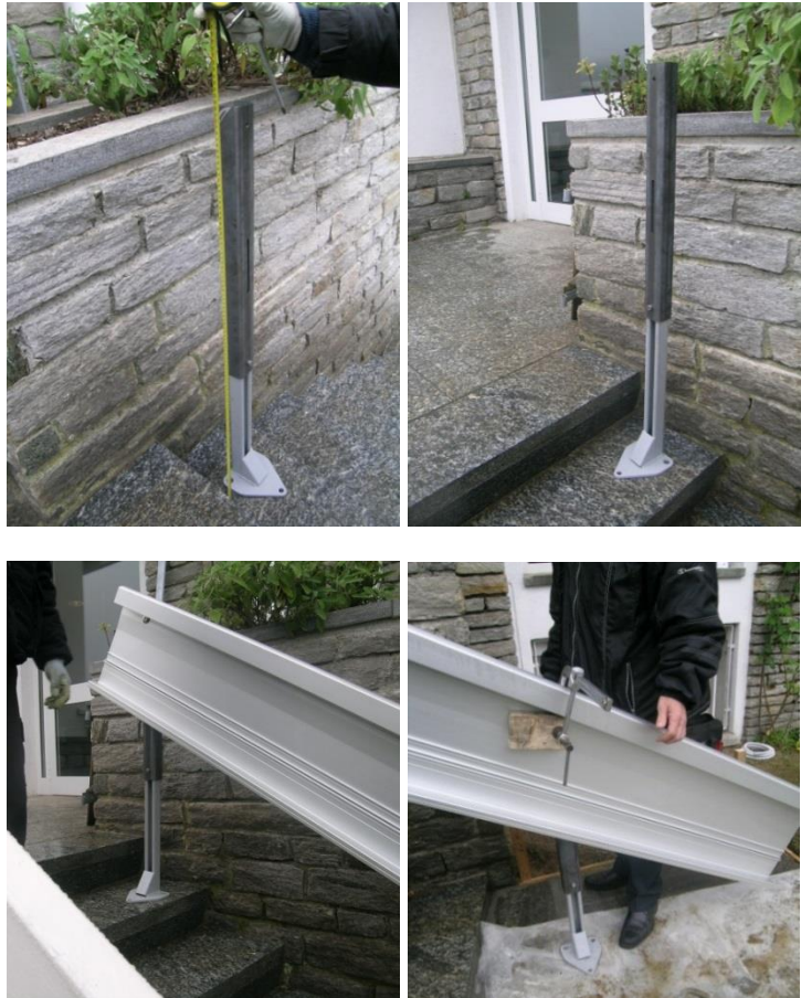
Fig. 3 – Positioning, adjustment and securing of the feet to the end of the guide
