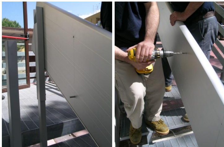
Fig. 6 – Detail of drilling the marked holes
