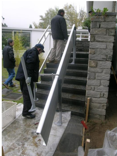
Fig. 4 – Positioning of the guide at mid stair
