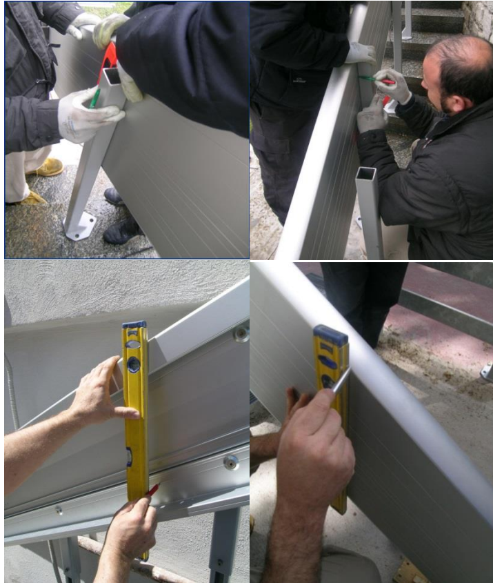
Fig. 5 – Various methods for marking the holes
